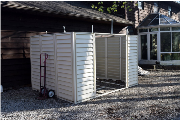
The 8 x 10.5 ft. Duramax Woodbridge shed with the walls up.
